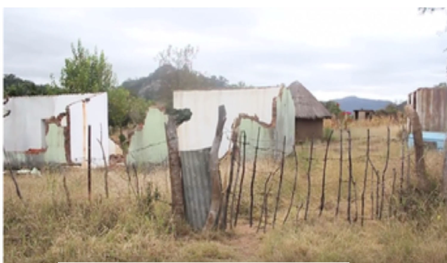
Demolished housing before displacements made of brick wall and cement
