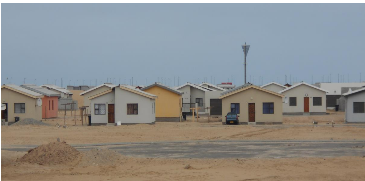
Figure 3: Houses built in Walvis Bay as part of the Mass Housing Development Program.
